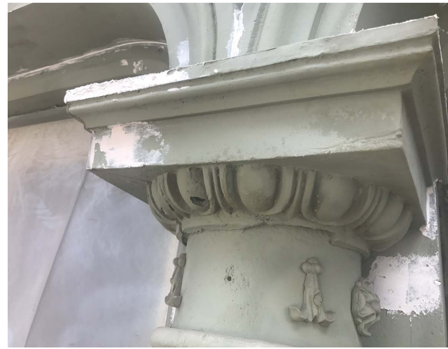
CRACKED COLUMN CAPITAL W/ MISSING ORNAMENTS
