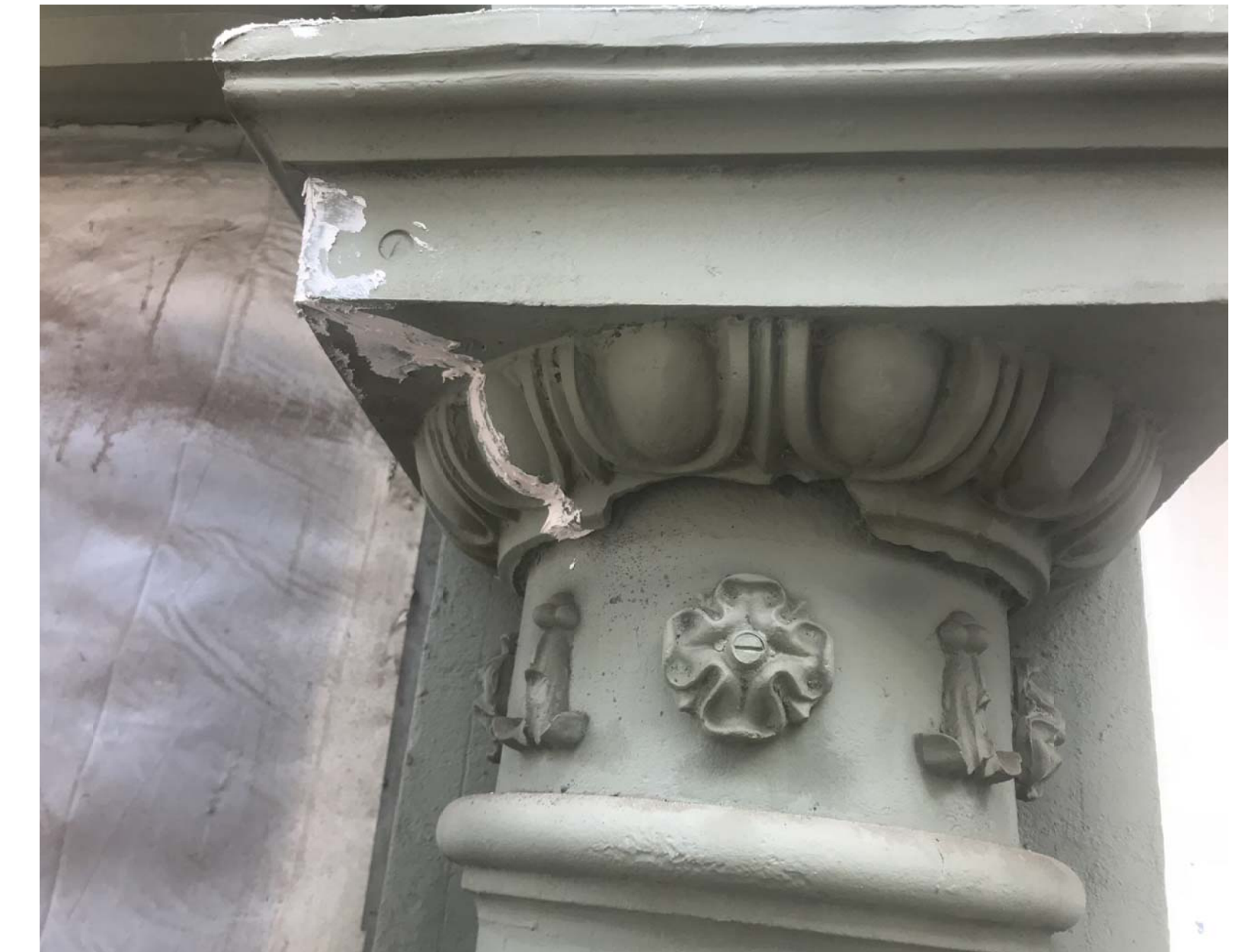
CRACKED / BROKEN C.I. COLUMN CAPITAL
