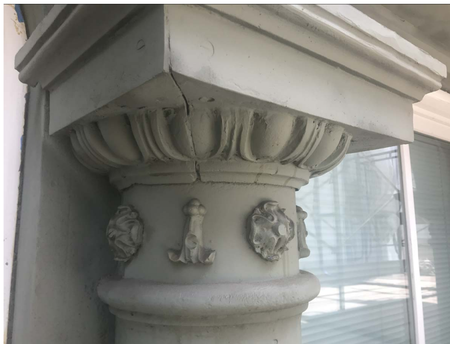
CRACKED C.I. COLUMN CAPITAL
