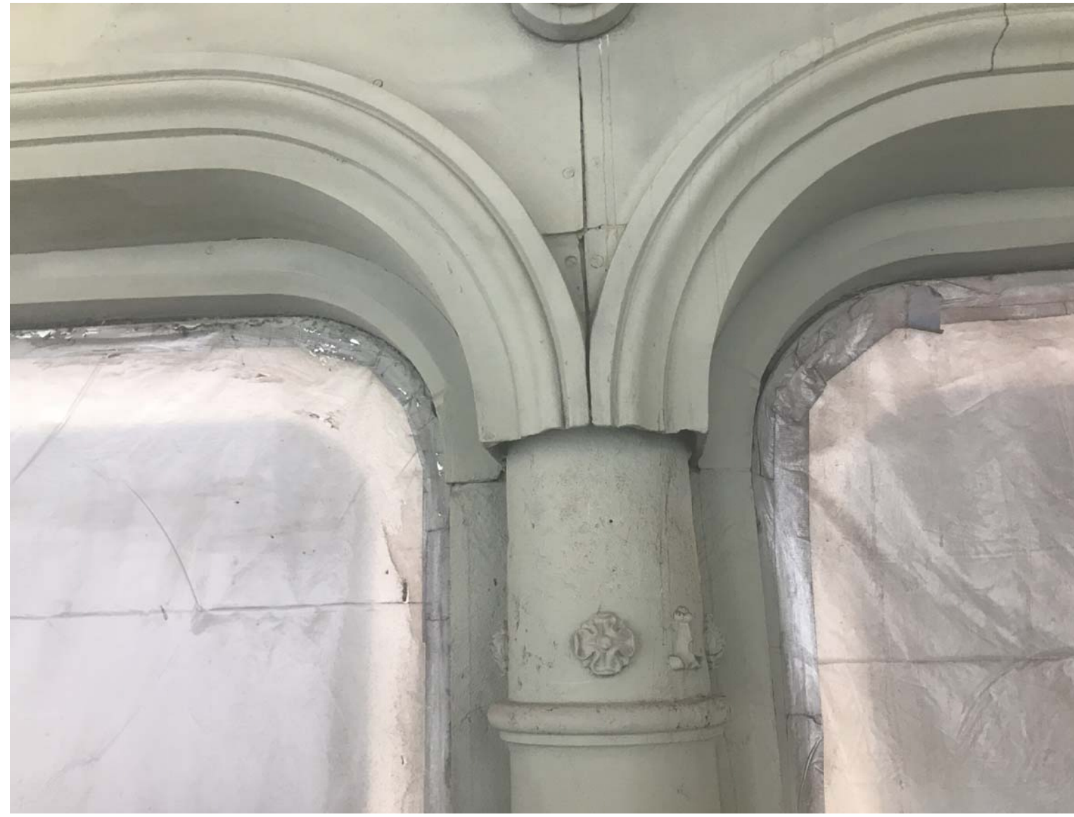
MISSING C.I. COLUMN CAPITAL
